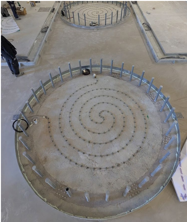
Fiber in place.
