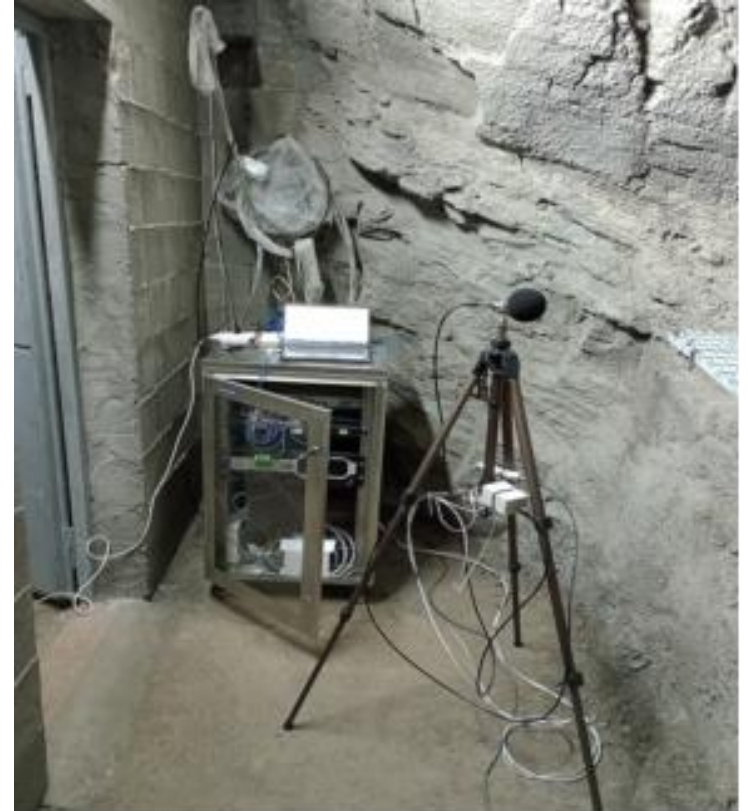
SOE1 Underground station
