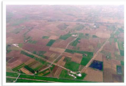
Aerial view of the site construction near Cascina (Italy)
