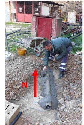
Few weeks ago, by taking advantage of the works for the water drainage in P2 and P3, the installation of the vertical magnetometers was prepared;
