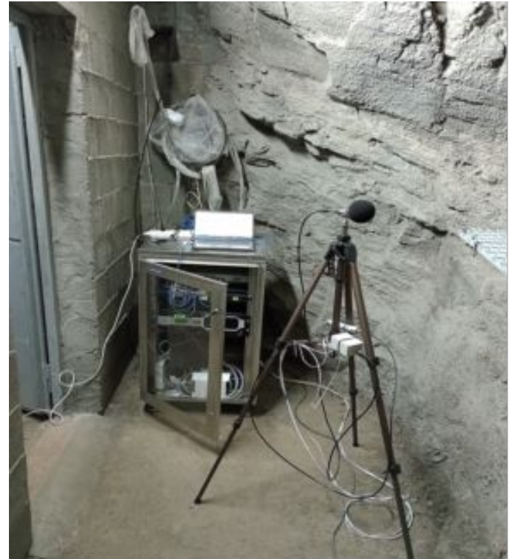
SOE1 Underground station
