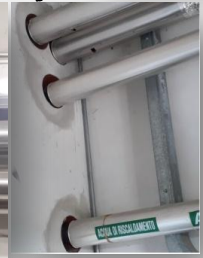
Through-holes in the wall
