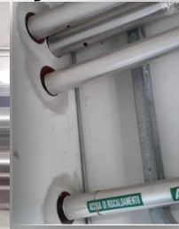
Through-holes in the wall
